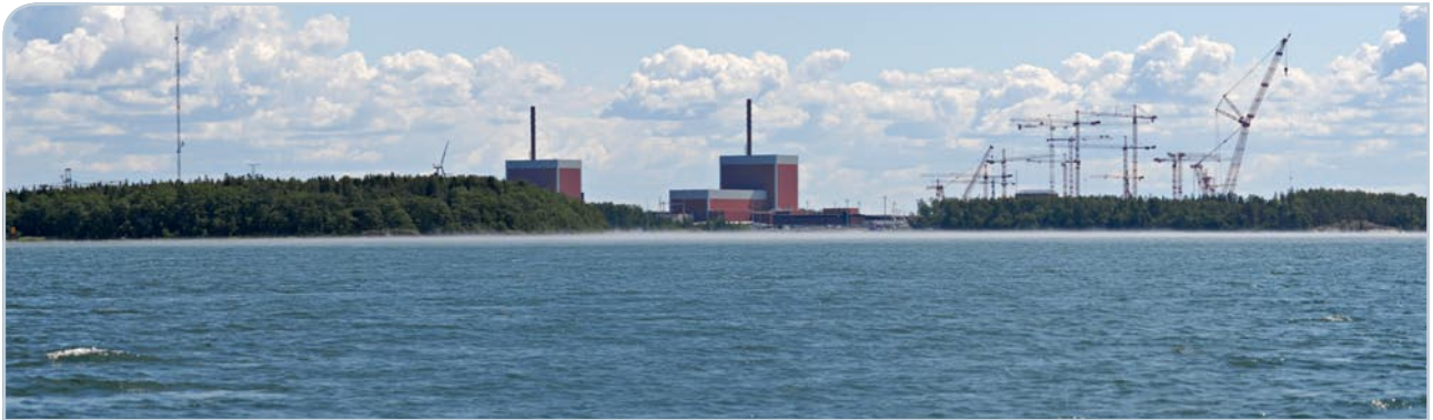
Figure 6. The nuclear power plant site of TVO as seen from the sea. The picture on top shows the existing plant units OL1 and OL2 and the OL3 construction site. The bottom picture is a photomontage that shows the existing plant units OL1 and OL2, the completed OL3 and OL4 on the left.
