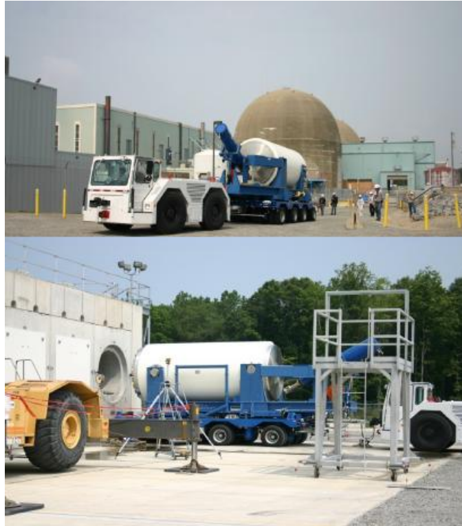
Fig. 20 NUHOMS system at the Metsamor NPP (AREVA, 2011)
