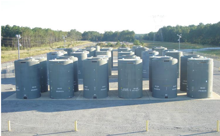
Fig. 32 HI-STORM 100 at the ASCO NPP (Holtec, 2013)
