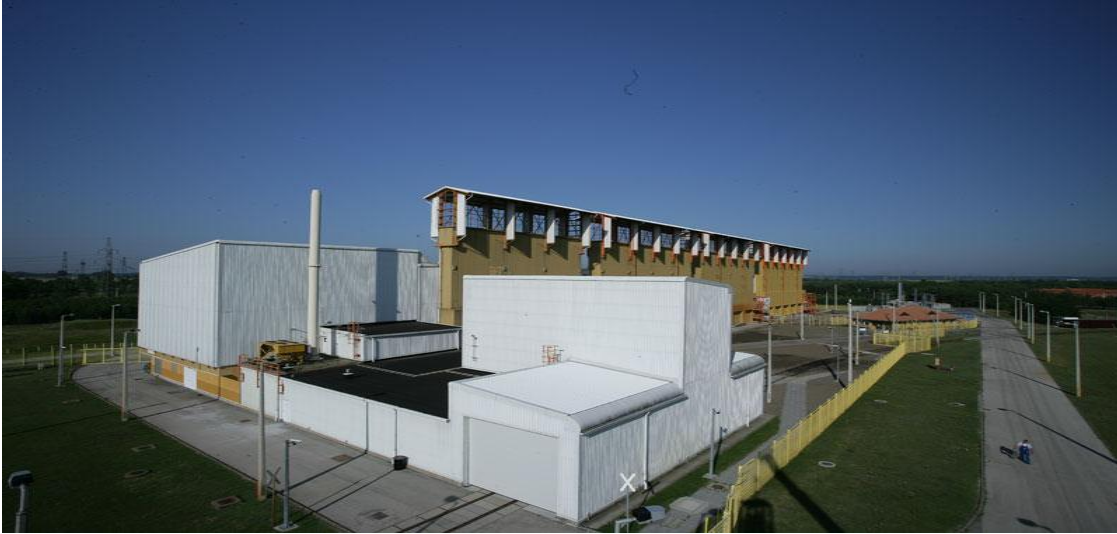
Fig. 8 Complete storage facility at the Paks NPP (RHK, 2009)
