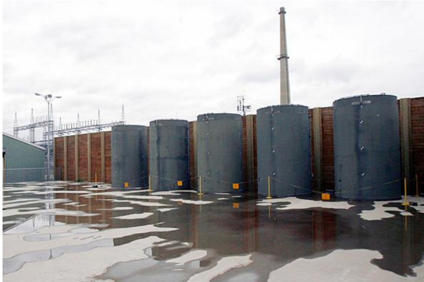
Fig. 12 Open interim storage facility at the Vermont Yankee NPP (Toby Talbot/AP/File, 2010)
