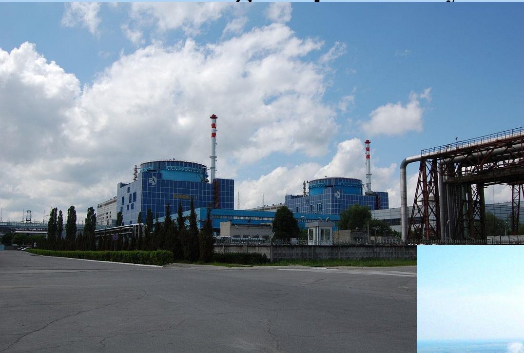
Khmelnytsky NPP, power unit №2, VVER-1000
