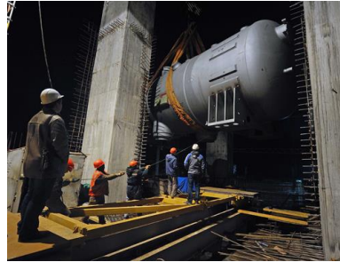
Steam generator installation at Leningrad-II-1
