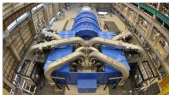
Siemens turbine (up) and Alstom turbine (down)
