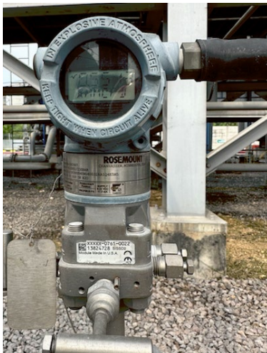
The compact orifice plate flow meter for lean gas (Rosemount 3051CFC )
