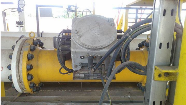
The Ultrasonic flow meter for feed gas/at Point F (Elster Instronmed Q. Sonic 4C)
