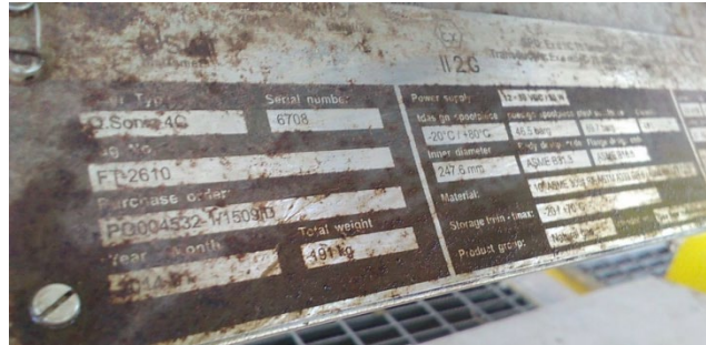
The Ultrasonic flow meter for feed gas/at Point F (Elster Instronmed Q. Sonic 4C)
