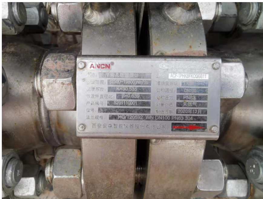
Image 3: The Orifice Plate flowmeter at point F
