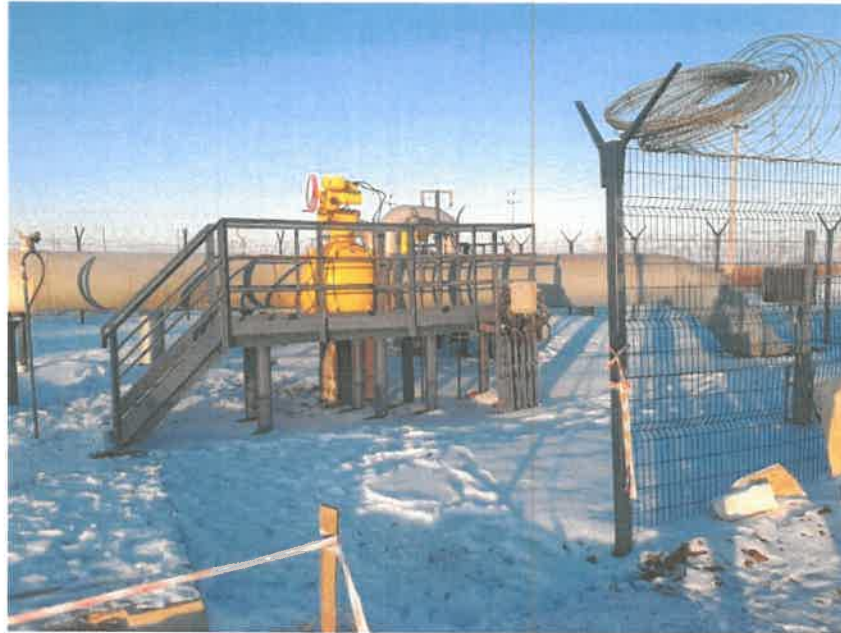
Figure C: New DN700 Pipeline
